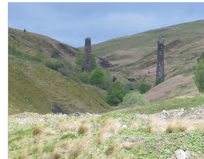
Glenbuck Viaduct, the remnants of a long lost village and strong socialist heritage of the area © Richard Webb (cc-by)
