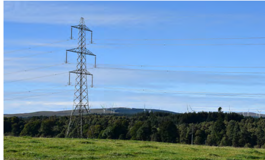
Work with ScottishPower Energy Networks to design an efficient grid network which is fit for the future © LUC
