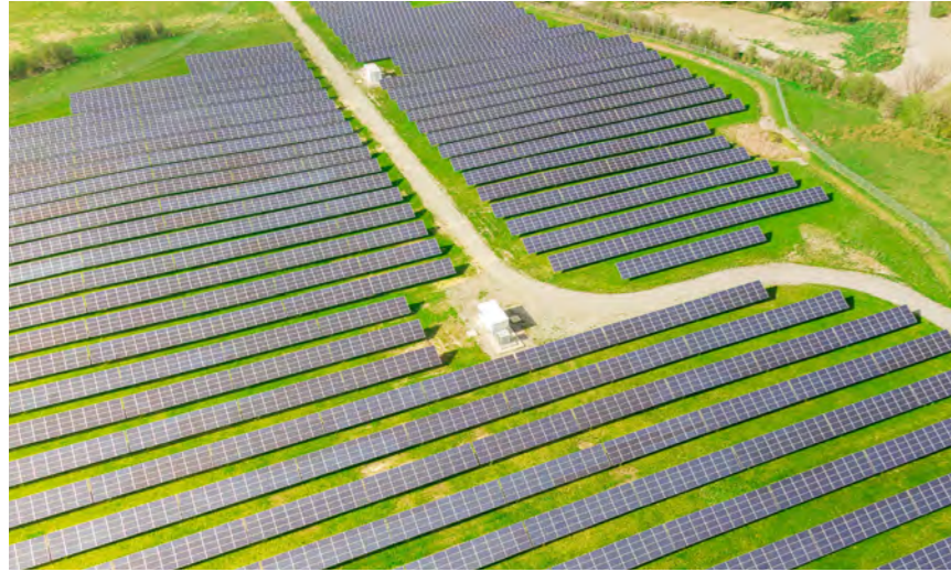
Co-location of solar PV (similar to the above) and energy storage technologies on appropriate sites across the cluster © LUC
